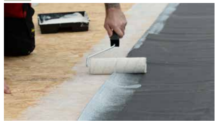
External roof covering is made from 1.2mm thick EPDM black rubber which creates a maintenance free waterproof membrane.
